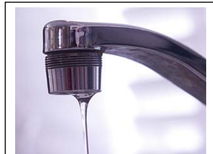
During extremely cold outside temperatures, turn faucets on to a slow trickle to reduce the chance that water lines from freezing.
